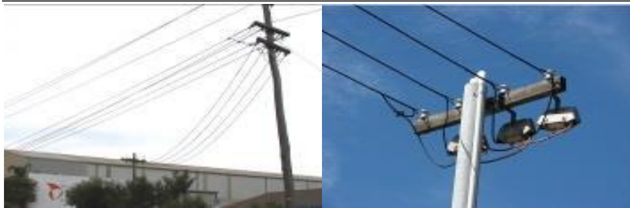
Figure 2: Larger than standard supply - overhead three-phase (bare)
