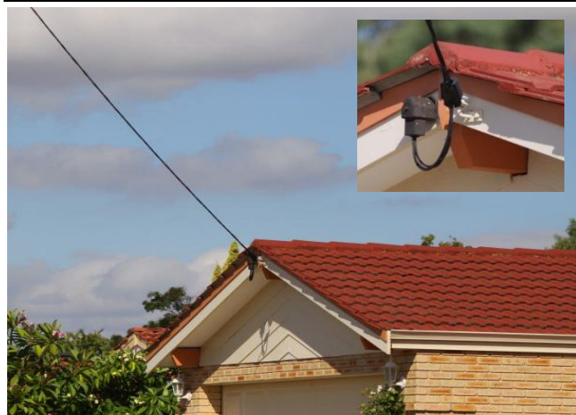
Figure 2: Larger than standard supply - overhead three-phase (bare)
