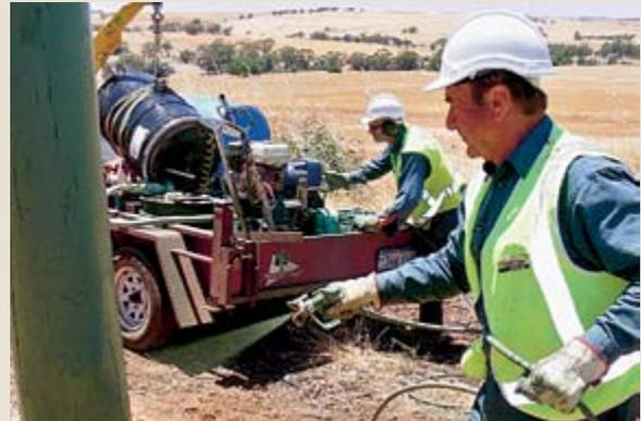
Western Power has started a program using fire retardant paint on all new wooden poles installed in regional Western Australia. The paint has been extensively tested and found to stop poles catching fire during low intensity fires such as scrub, brush and grass fires.
