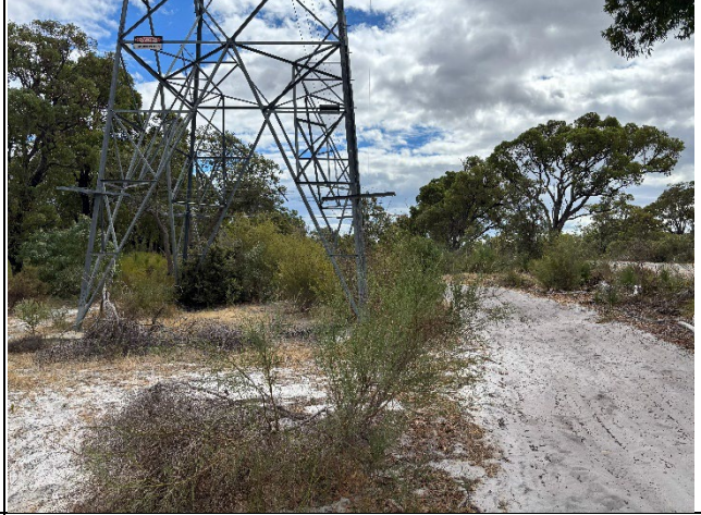
Photo 6 – Wesco Road existing maintenance corridor
