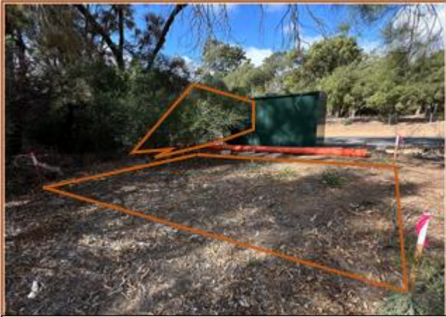
Image 2: Clearing area #1 (marked in orange) to facilitate new RMU.
