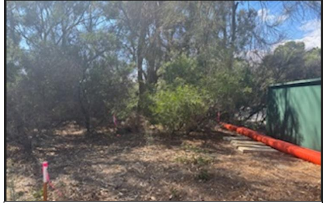
Image 3: Photo of new RMU location and vegetation clearing area.
