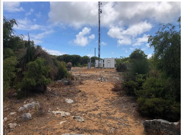
Photo 4: Photo showing the cleared area around the stays heading back to the fire protection zone.
