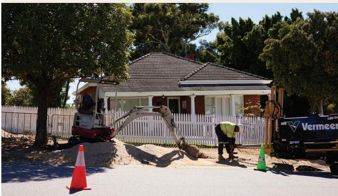
*Digging an entry/exit hole for a drill shot.*
