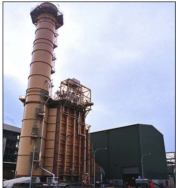
Above - Cockburn One Power Station.
