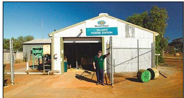
Above - In the Mid West town of Yalgoo, the old diesel-fired power station closed on 17 November 2003.
