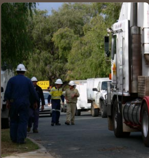
Restoring power after the Clarence Street Substation fault.
