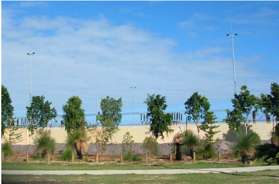
At completion (April 08)
