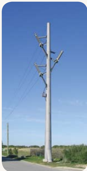
132 kV steel transition structure.
